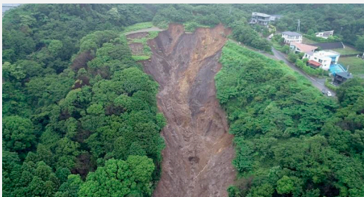
Embankment collapse at the head of Aizome River Shizuoka Prefecture UAV photograph (July 3, 2021)
